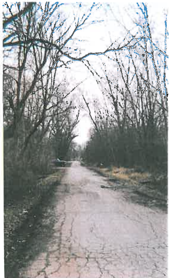
South Shore area street in poor condition
