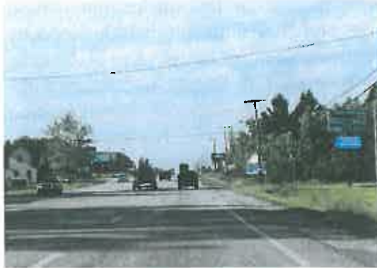
US Highway 41 Traveling South into Cedar Lake from US Highway 231
