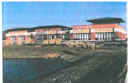
Example of a High-quality Office Park
