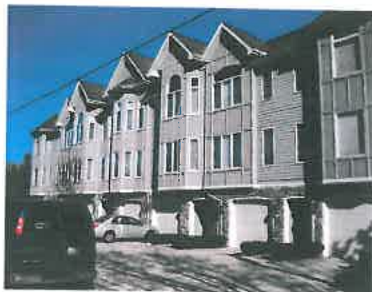
High Density Residential units along Cedar Lake
