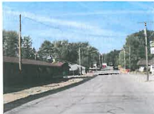
North Laked-shore Drive is one (1) of several minor arterial streets in Town.
